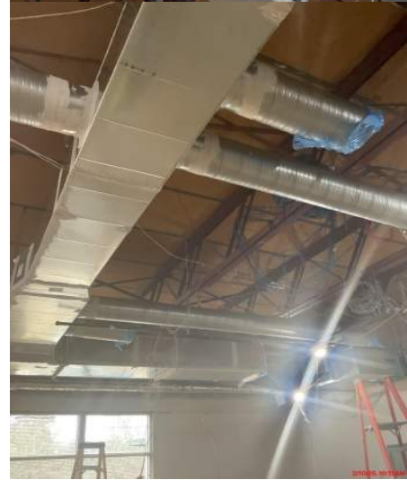
Continue installing ductwork in cafeteria
