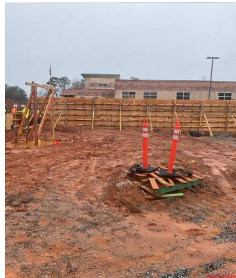
Wall foundation formwork in place.
