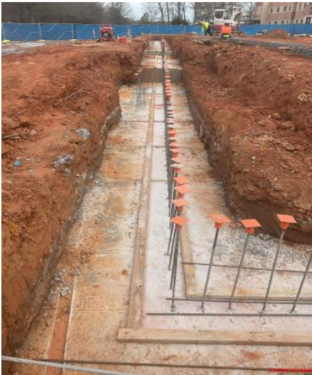
Footing poured per gridlines 4 and D
