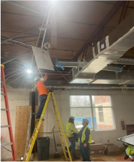
Conduit for gym feeders & cafeteria lighting rough-in
